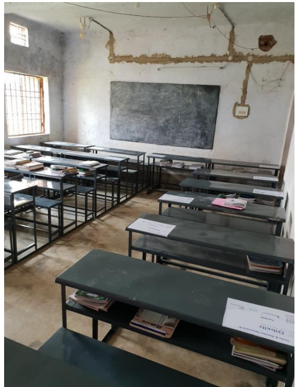
New tables and benches for the classroom. The newly laid power lines can be seen above the blackboard.
